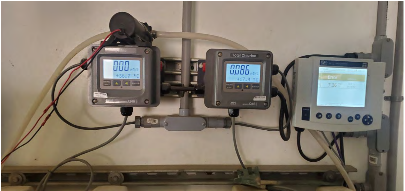
Figure 6: Total chlorine and bisulfite analyzers located at the effluent discharge building. The Facility was not discharging to surface water at the time of the
