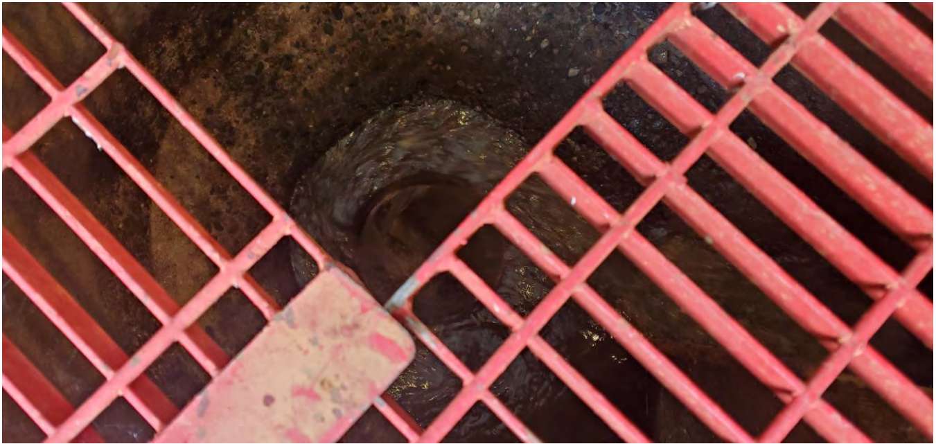
Figure 2: The influent goes through a comminutor to shred large solids before being pumped to the aerated treatment pond.
