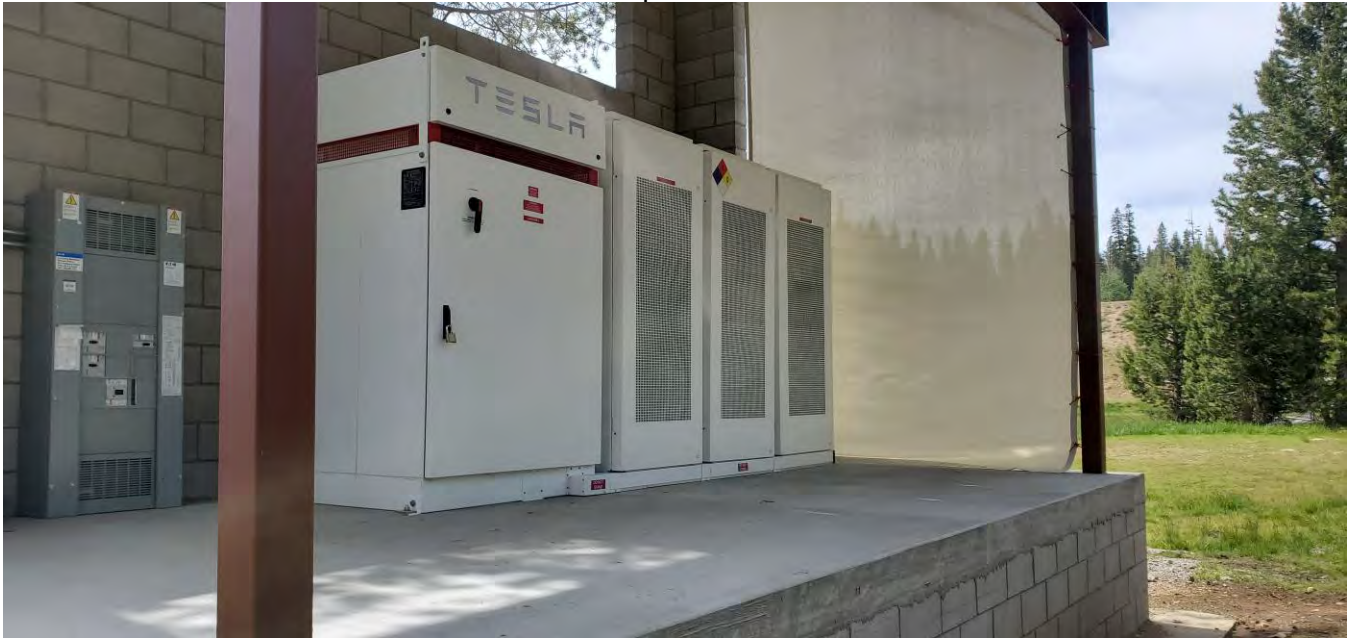
Figure 6: The newly installed Tesla battery pack for emergency power generation.
