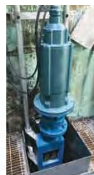
This grinder is utilizing a submersible (IP68) motor.
