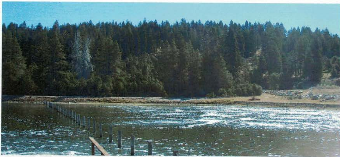
Figure 3: The 12.5 million gallon treatment pond is aerated through diffusers located at the bottom of the pond.
