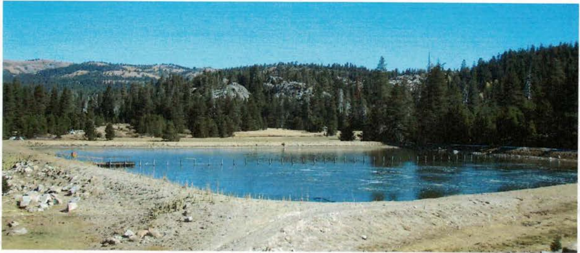
Figure 3: The 12.5 million gallon treatment pond is aerated through diffusers located at the bottom of the pond.
