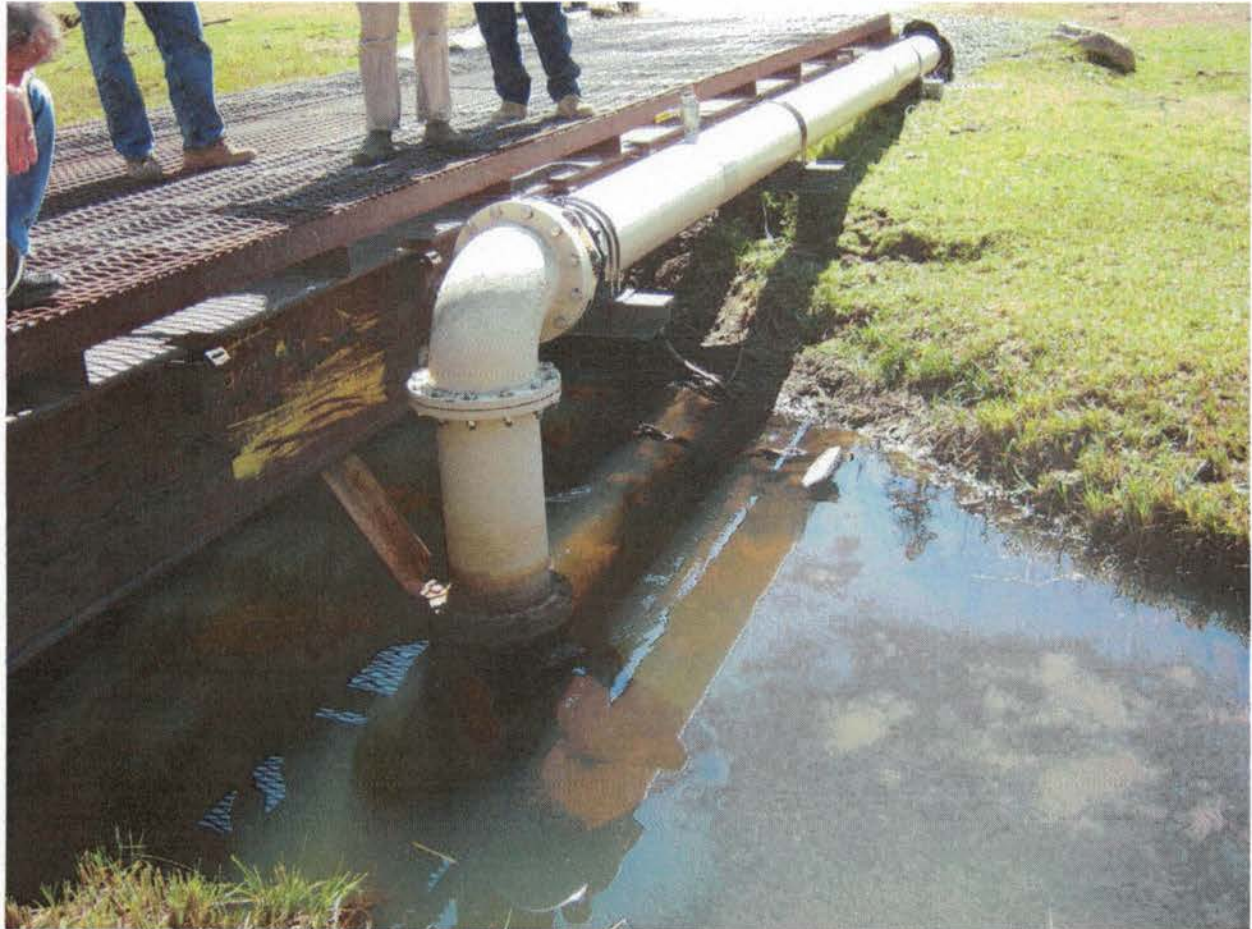
Figure 2 - Effluent Outfall in Bloods Creek
