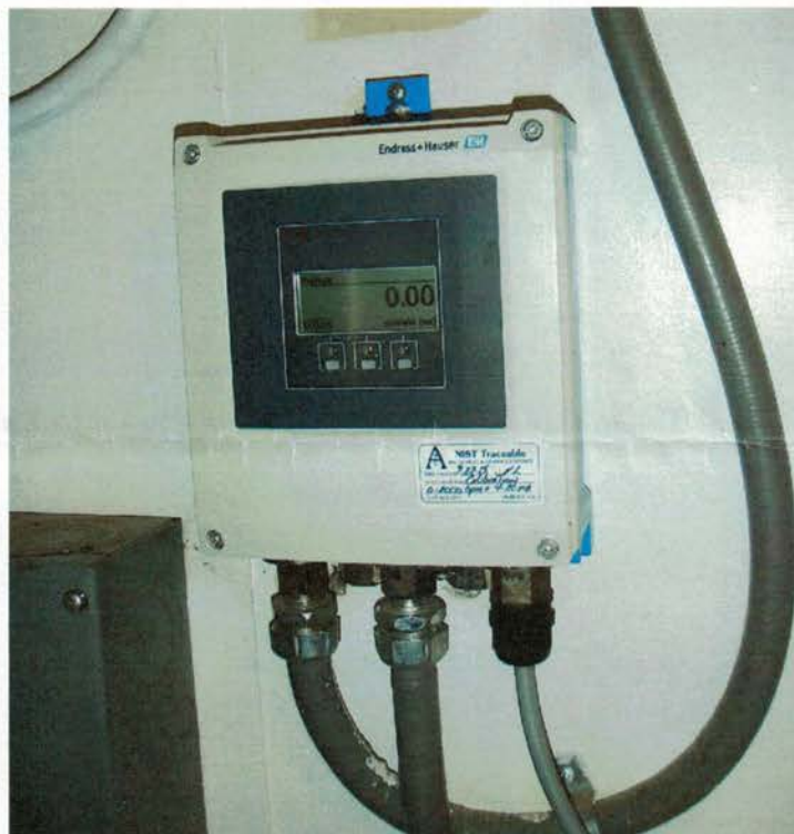
Figure 6: The effluent flow meter. The Facility was not discharging to surface water at the time of the inspection.
